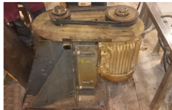
↑ Oven Re-Circulation Fan Unit
